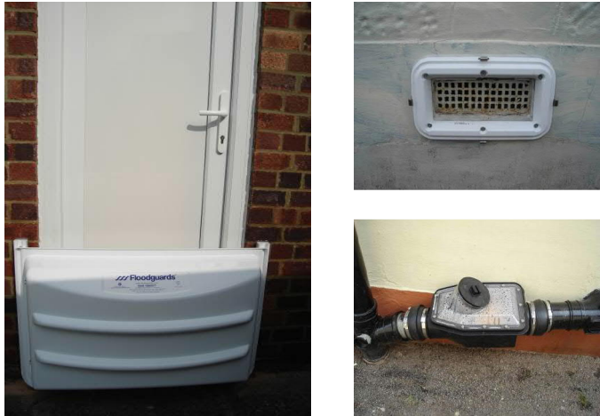
Figure 5-3 Examples of flood barriers, air bricks and on-return valves
