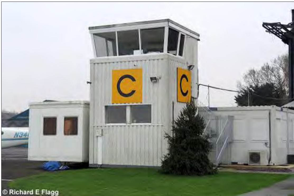
Figure 9 – ATC Tower at Elstree Aerodrome
