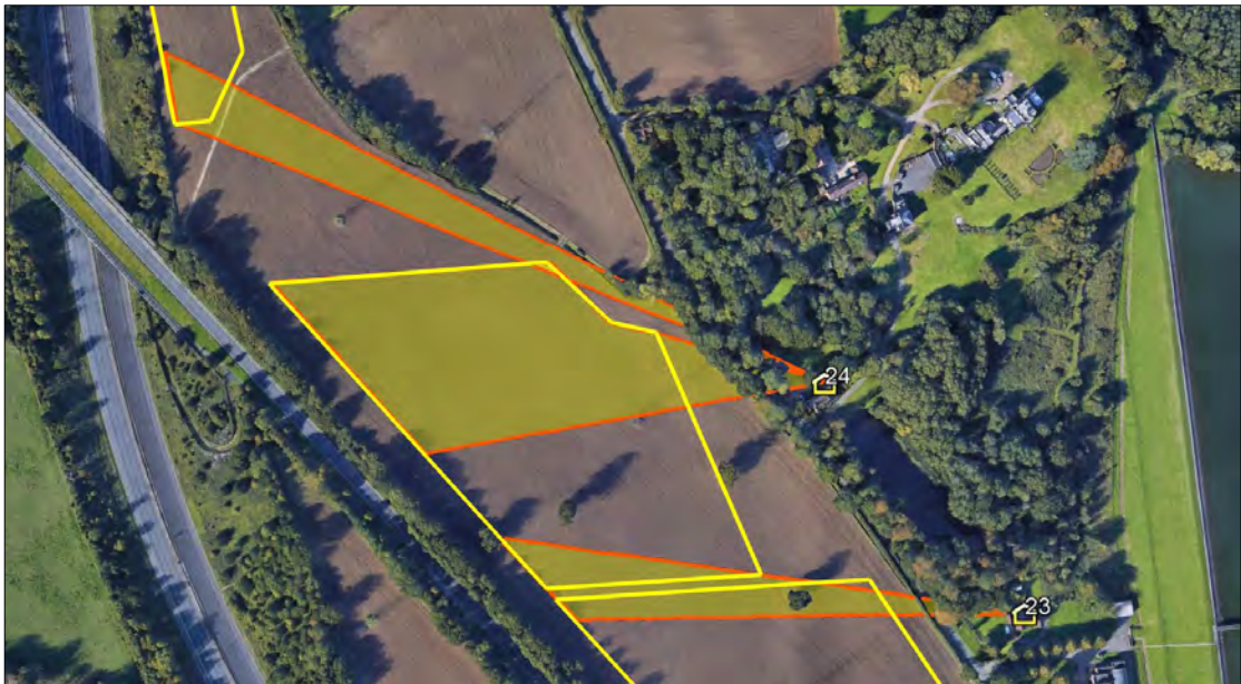
Figure 33 – Location of dwellings 23 and 24 relative to the reflective area and level of screening
