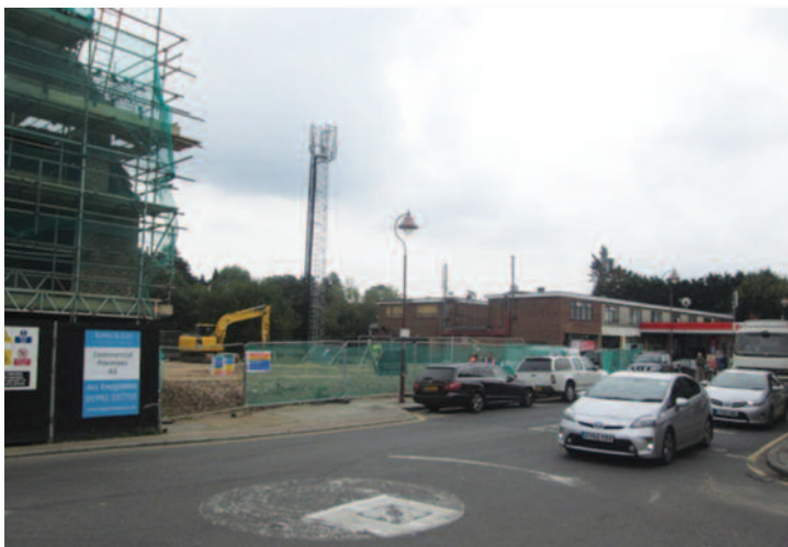
Photograph 2: The former Radlett Fire Station (recently demolished) viewed from the west
