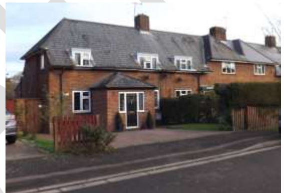
Figure 2.24: Using a half hipped roof can reduce the bulky appearance of living space within the roof compared with a gable or crown roof.
