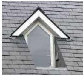
Figure 2.26: A recessed dormer ( http://www.builderbill-diy-help.com/dormer-
