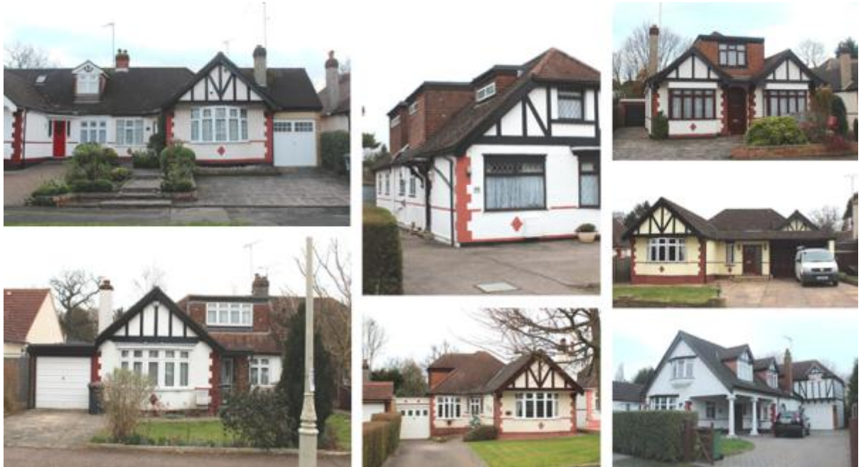
Figure 9 Examples of inappropriate alterations
