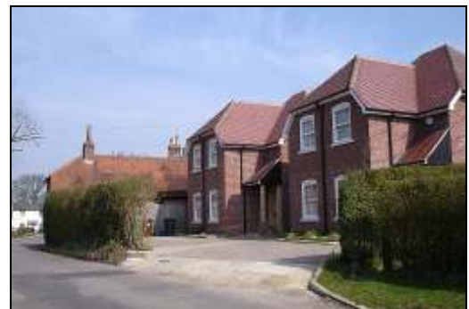
New development with unresolved threshold to street. Pound Lane
