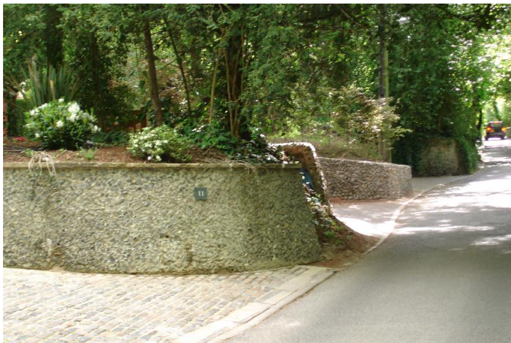
Figure 11. Flint walls on Loom Lane.
