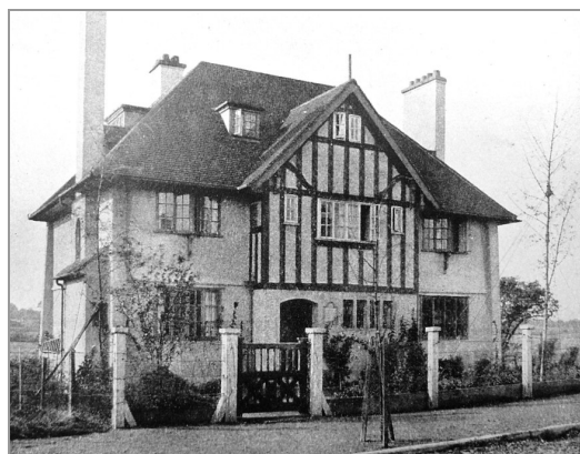
Photograph of Homeleigh , The Avenue (front)
