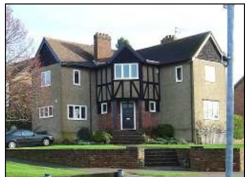
33 The Avenue, a winged-house type; one of the original 1920s houses
