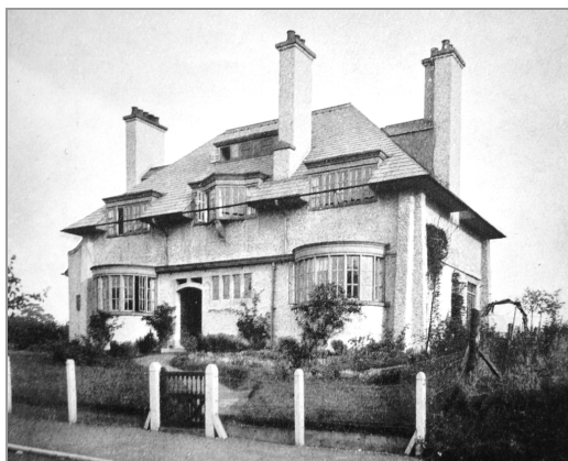
Photograph of Seldown , The Avenue (front)
