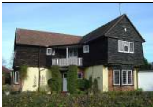
3 The Avenue, a winged-house type; one of the original 1920s houses
