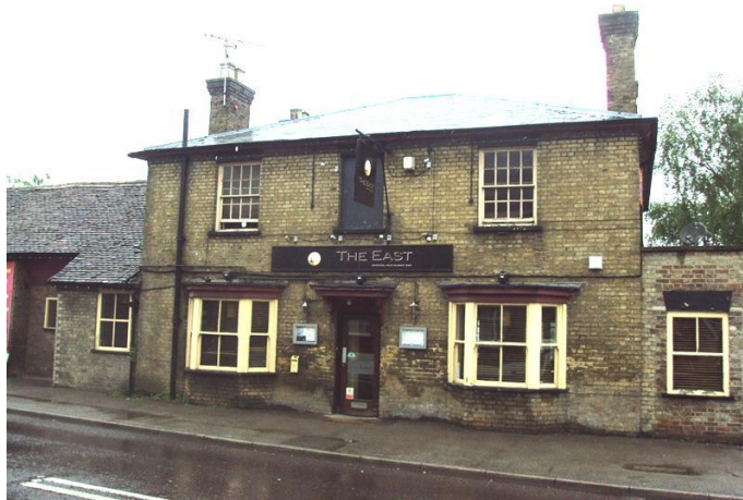
Figure 11: The East restaurant (former Plough Inn), High Street (Above)
