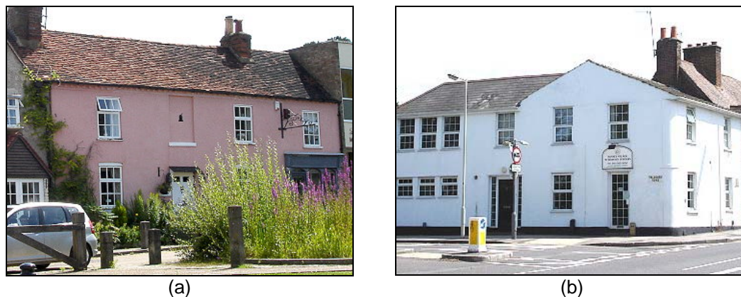
Figure 20. Character Zone 1: loss of traditional architectural features; replaced doors and windows in the High Street, Prospect Cottage (a) and No. 2 (b)
