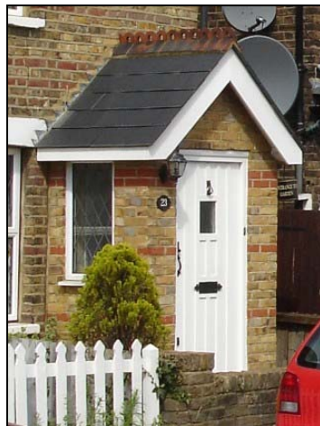
Figure 41. Character Zone 3: loss of traditional features; (top) pebble dashing to exposed brick walls & sash windows replaced with modern casements; (bottom) two similar examples of added porches. The brick type and red brick detailing used on the porch to the left has tried to match the external detail of the house, compare to the porch on the right.
