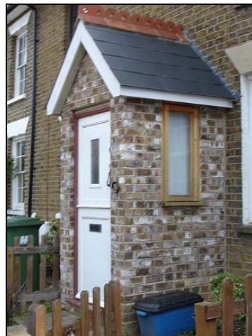
Figure 41. Character Zone 3: loss of traditional features; (top) pebble dashing to exposed brick walls & sash windows replaced with modern casements; (bottom) two similar examples of added porches. The brick type and red brick detailing used on the porch to the left has tried to match the external detail of the house, compare to the porch on the right.
