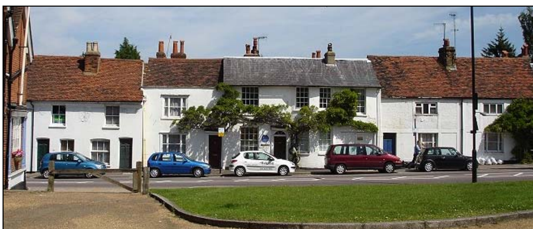
Figure 16. Character Zone 1: views; vernacular-style whitewashed cottages on the north side of the High Street (nos. 16 - 22)
