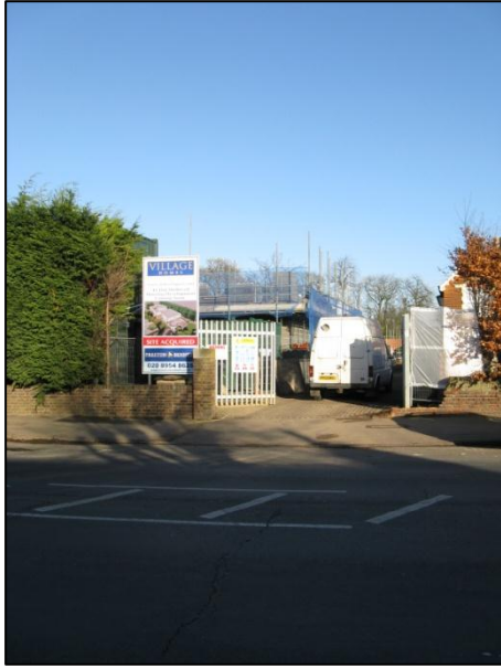
Figure 16 - Entrance point to redevelopment to the rear of High Road.
