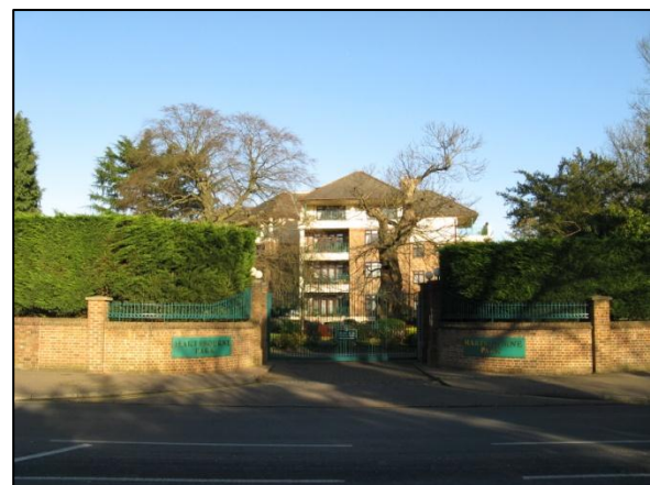
Figure 31 - The main entrance of Hartsbourne Park
