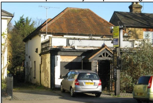
Figure 35 - The former Devonshire Arms.
