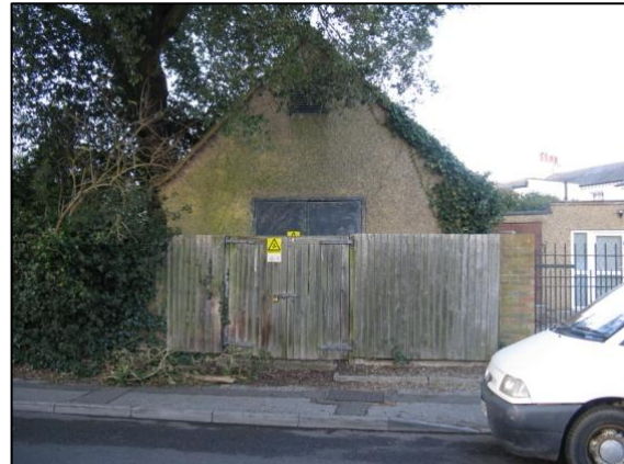
Figure 27 - The electrical substation along Hartsbourne Road.
