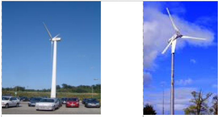
Figure C1: Freestanding wind turbines, Vestas V29 225kW wind turbine at Beaufort Court, RES Ltd in Hertfordshire (left) and Proven 15kW wind turbine (right)
