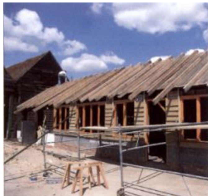
Conversion of farm building
