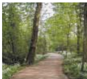
The completed Greenway at Allum Lane Spinney
