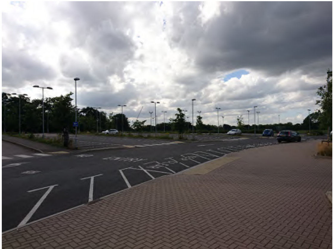
Photograph 3 Car park at Bushey Academy, in the south-west corner of the parcel
