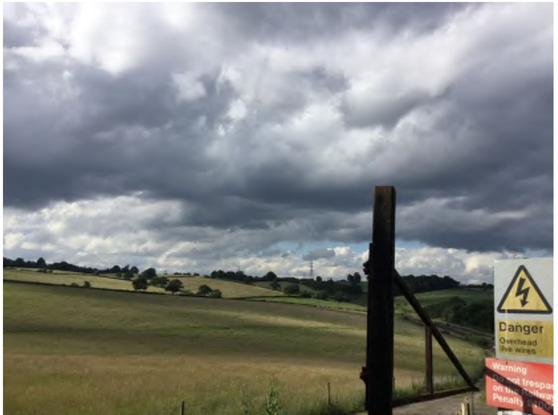
Photograph 3 Facing north across the parcel from Waggon Road, with the East Coast Main Line in the right of the shot
