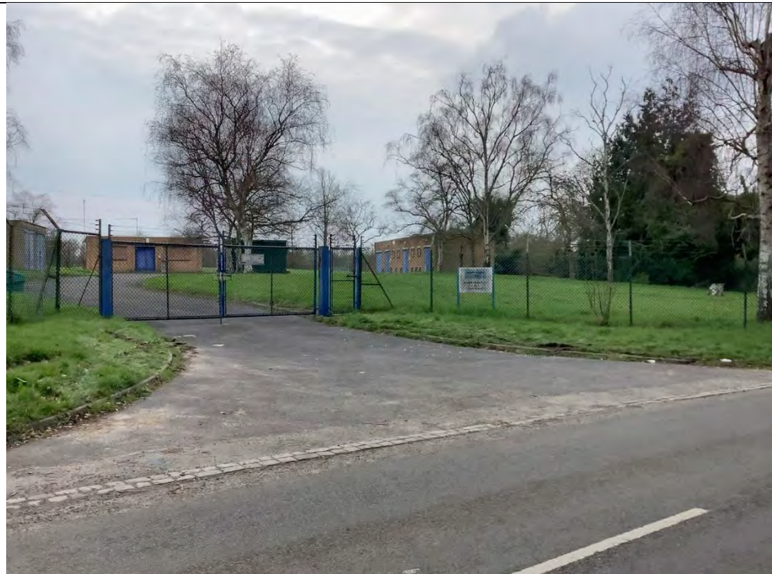
Photograph 4: View of facing south-west from Berry Grove Lane, showing view of utility sub-station.
