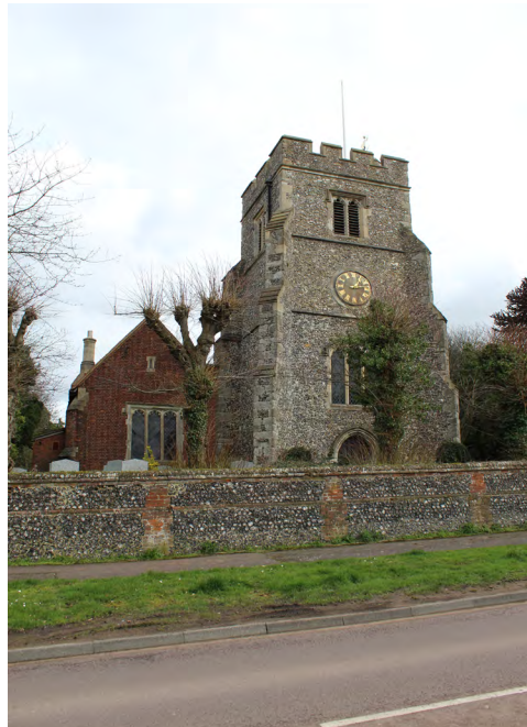
Figure 17 Flintwork of the tower of St Giles Church and church yard wall
