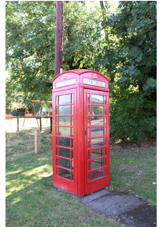
Figure 34 K6 Telephone Kiosk
