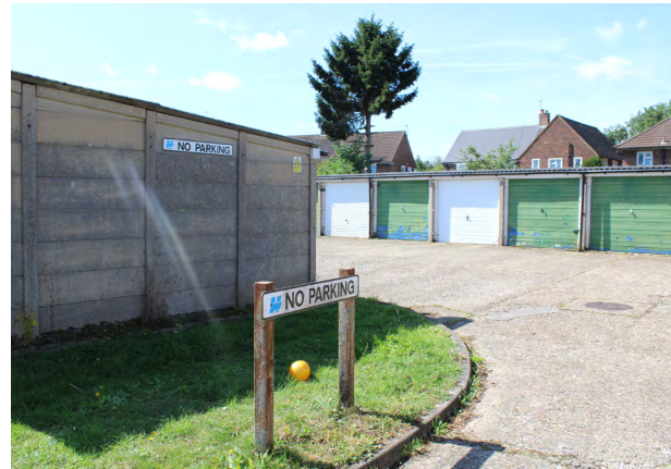
Figure 72 Garage site to the rear of South Mimms Village Hall
