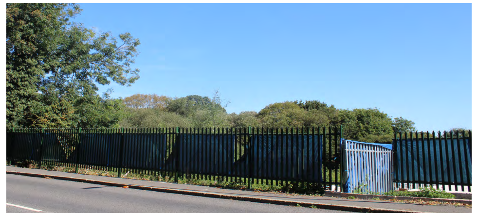
Figure 78 Metal railings on St Albans Road
