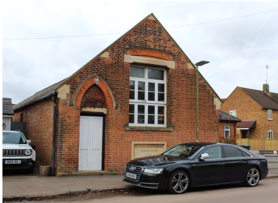
Figure 35 South Mimms Village Hall (Parish Rooms)
