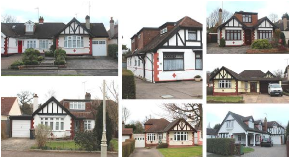
Figure 9 Examples of inappropriate alterations
