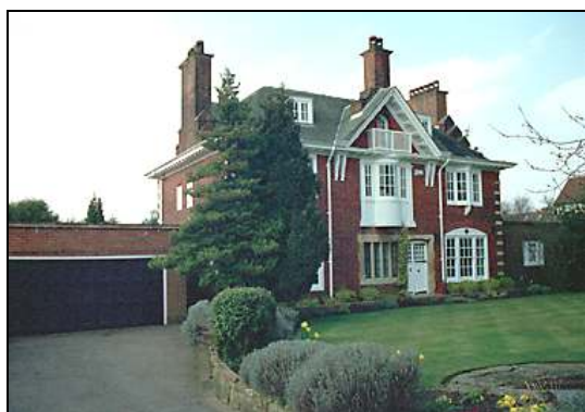
'Tiverton', Darkes Lane. 1908. Listed building (photograph taken from the English Heritage website: www.imagesofengland.org.uk )
