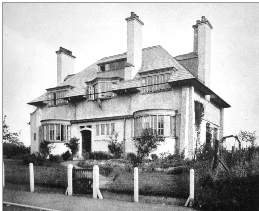
Photograph of Seldown , The Avenue (front)
