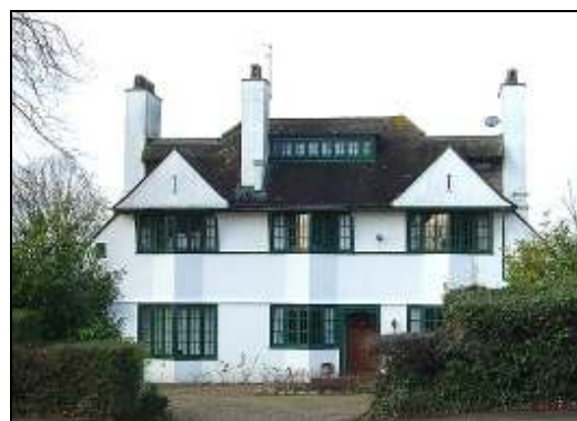
'Chestnut Tree House', Darkes Lane. 1908. Locally listed building
