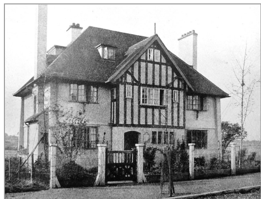
Photograph of Homeleigh , The Avenue (front)
