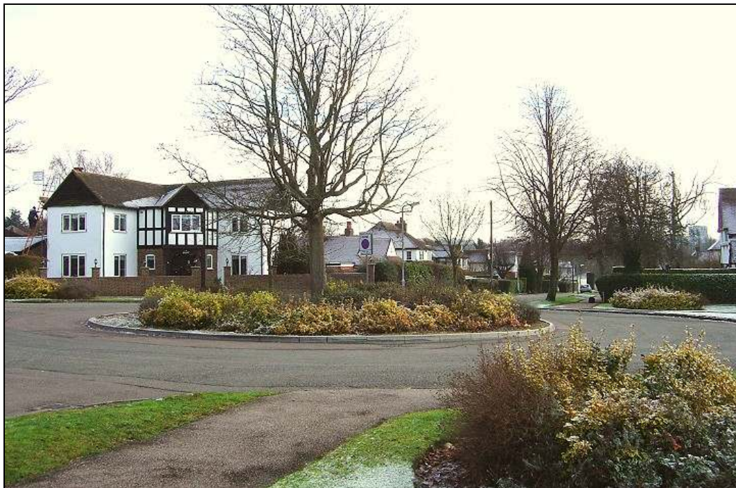
The same view of Heath Drive today. The photograph shows an example one of the four 'winged-houses' (no. 39 Heath Drive) that lie on each corner plot around the island. All survive and form a good group.
