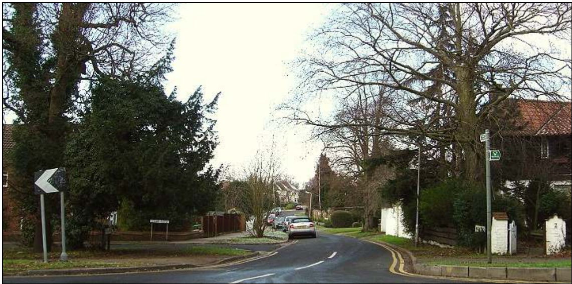
Mountway looking east from Darkes Lane (2 Darkes Lane, a winged-house type, is on the right)
