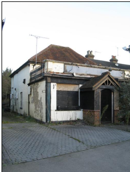
Figure 14 - The Devonshire Arms, now closed and dilapidated.
