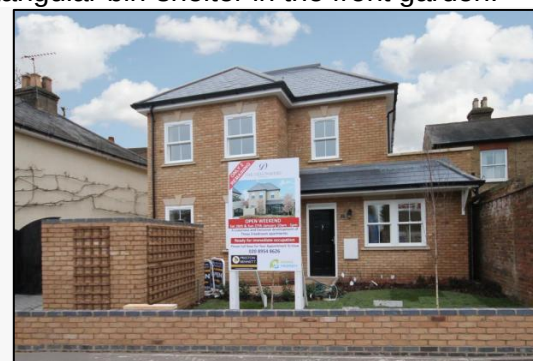
Figure 36 - The new 'Devonshire' development.
