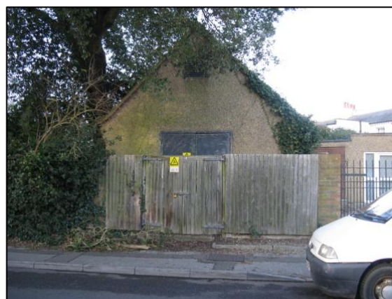
Figure 27 - The electrical substation along Hartsbourne Road.
