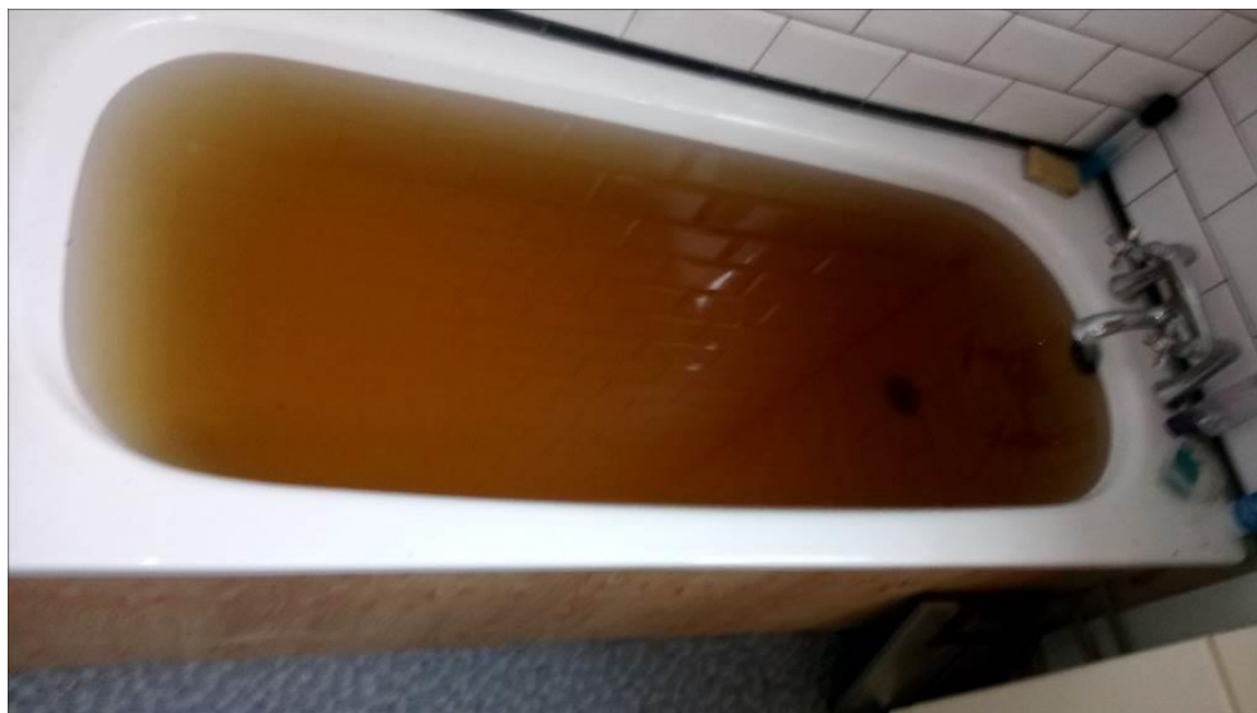
Figure 23: Extent of discolouration of water
