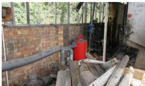
Figure 21: Supply pipework in an inadequate and unacceptable environment
