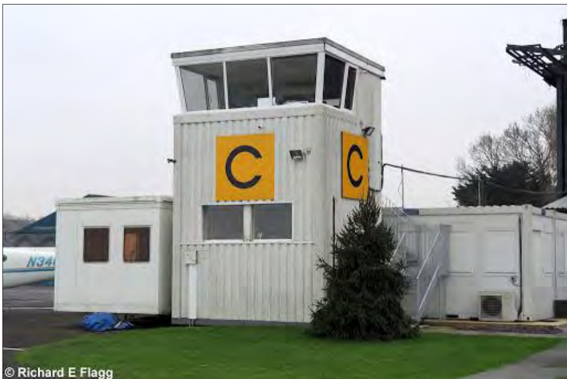
Figure 9 - ATC Tower at Elstree Aerodrome
