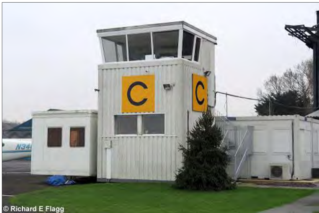
Figure 9 – ATC Tower at Elstree Aerodrome
