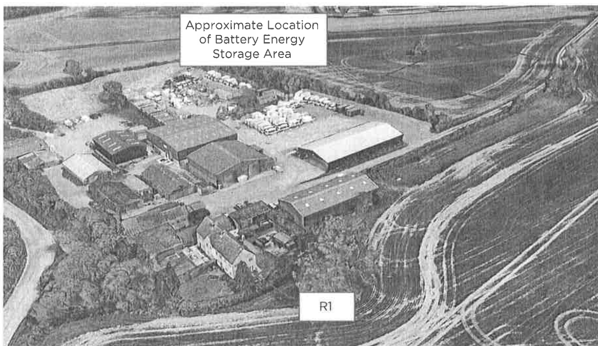
FIGURE 1: R1 AERIAL VIEW
