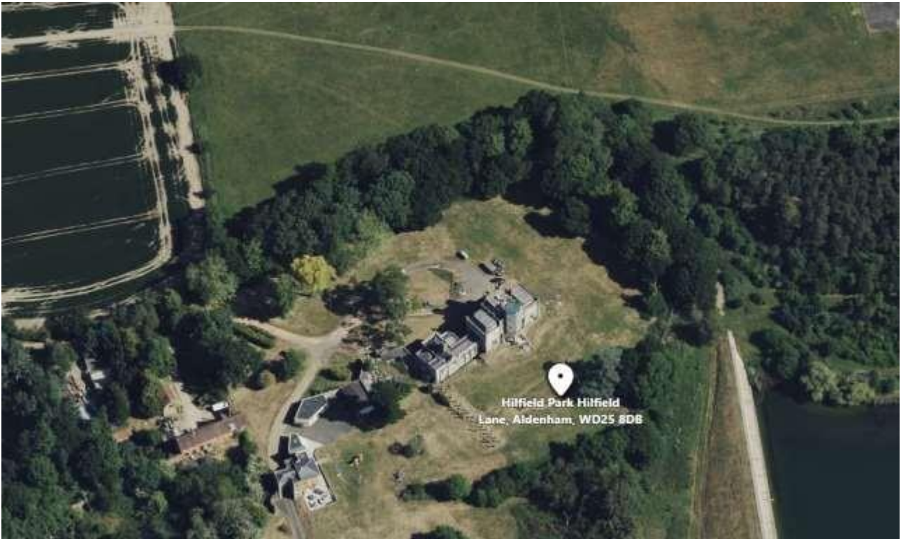
Figure 9 – Bird’s Eye view of Hilfield Castle (Bing Maps) looking generally northward. The disposition of trees is very different from the way it appeared in 1949 (Figures 7 and 8), with more emphasis on perimeter planting, and the formal gardens have been replaced with lawns. The Appellant seems to be relying on the density of the perimeter planting (which may be more visually permeable in winter months) in order to suggest that the solar array will only have a relatively small effect on the setting of the grade II* listed building. This does not take account of the fact that the present arrangement (gardens and perimeter planting) is already a departure from what would have been experienced historically, by the Villiers and Timins families, and, indeed, by other occupants well into the 20 th century. It may change again in the future.
