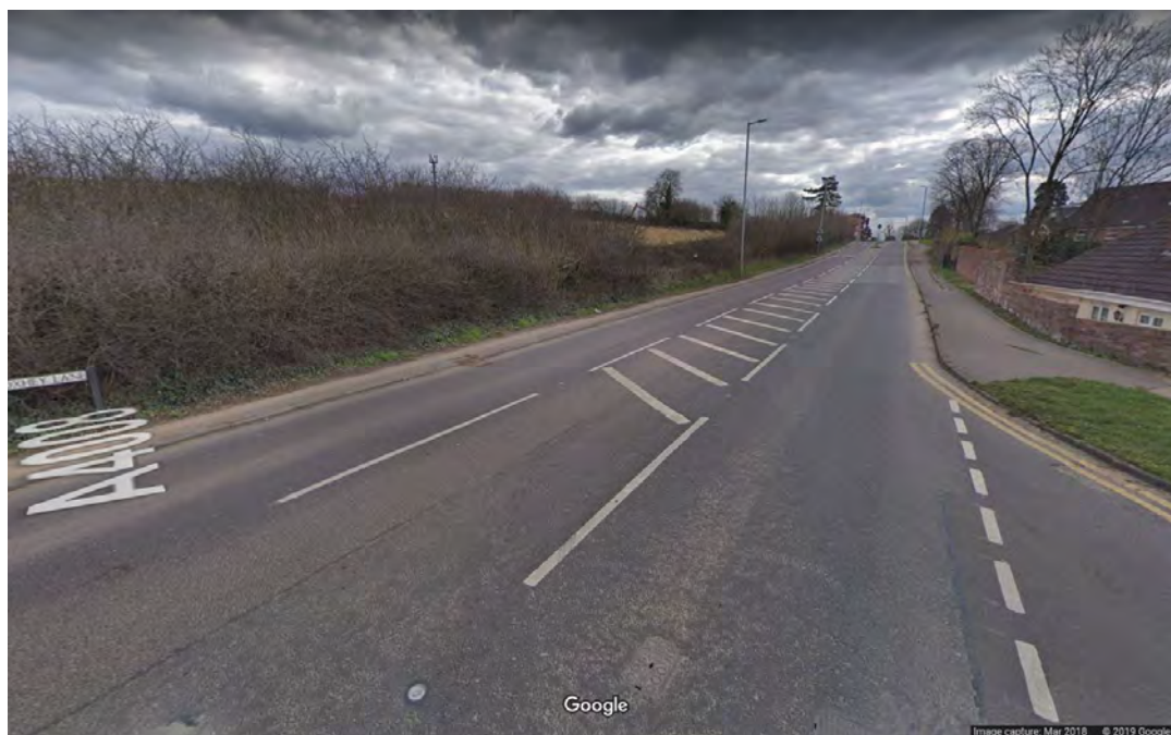
Existing visibility to the right from Carpenders Avenue onto the A4008
