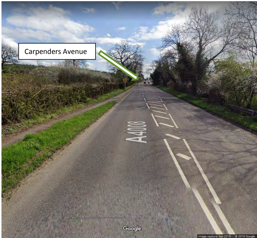
Southbound Forward Visibility to Carpenders Avenue (~130m)
