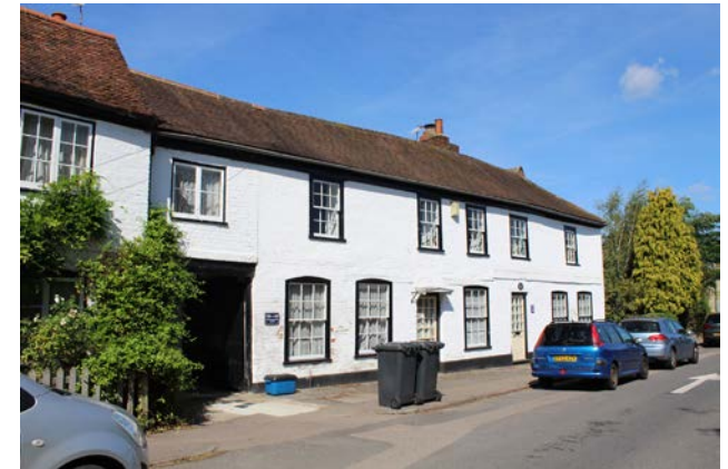
Figure 31 Painted brick elevations of 62 and 64 Blanche Lane
