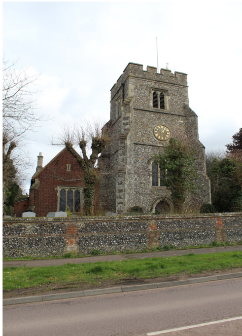
Figure 17 Flintwork of the tower of St Giles Church and church yard wall
