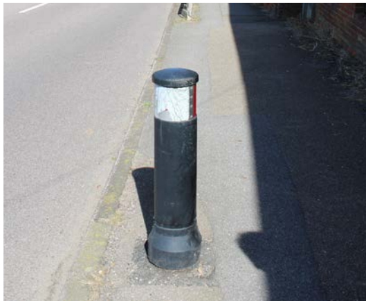
Figure 78 Plastic bollard on Blanche Lane
