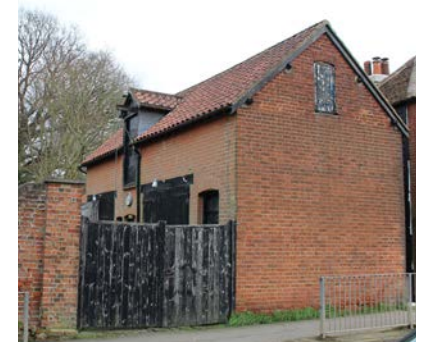
Figure 26 Former Vicarage stable and cartshed
