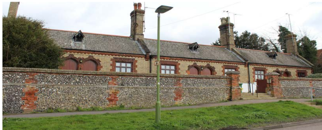
Figure 18 Gault brick and red brick dressings of Brewers' Almshouses
