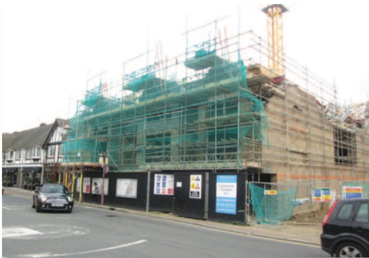
Photograph 3: Former Burrell & Co site viewed from the south west
