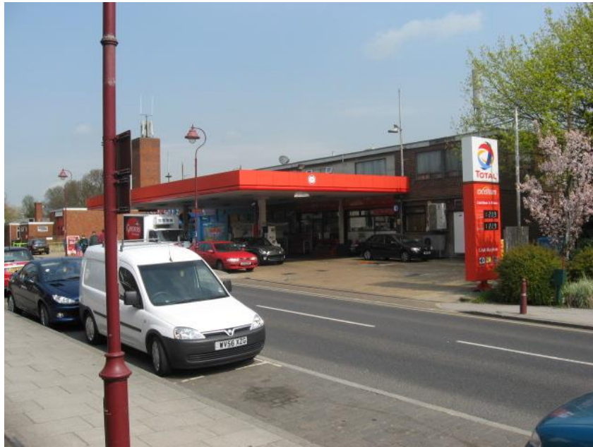
Photograph 1: Radlett Service Station/Regency House viewed from the south
