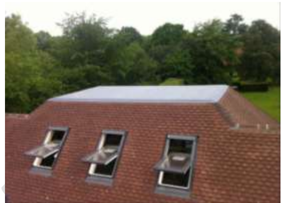
Figure 2.23: Example of a crown roof used to create additional habitable space in the roof.
