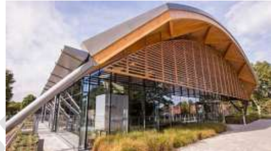
Figure 3.7: The WWF Living Planet Centre, Woking, uses double instead of triple glazing as it was more carbon efficient over the lifetime of the building.
