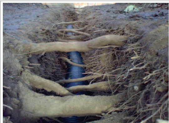
A section of drainage pipeline installed under tree roots following excavation using an air spade.
