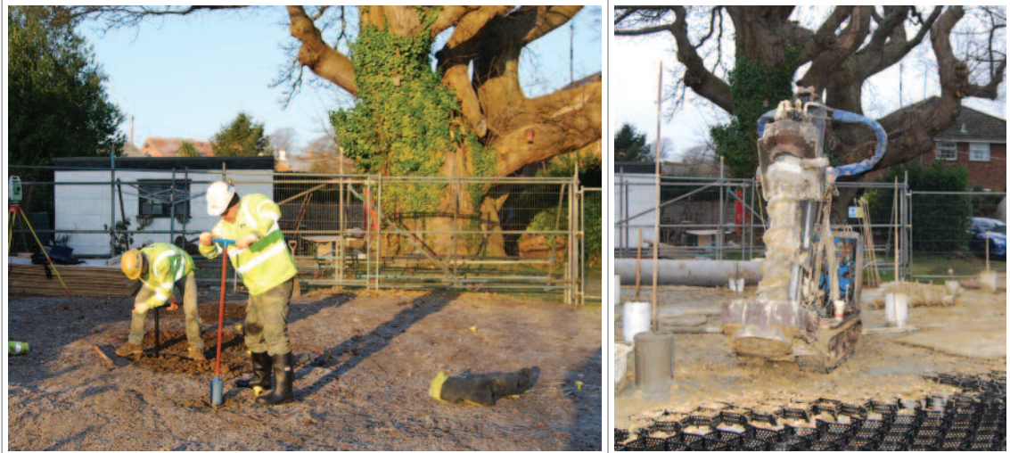
Using a hand auger to ensure proposed locations for piles do not conflict with tree roots within the root protection area of a veteran sweet chestnut tree. Note the BS 5837:2005 specification fencing in the background. The area was then covered with ground protection to allow a lightweight piling rig to work without damage to the underlying tree roots.
