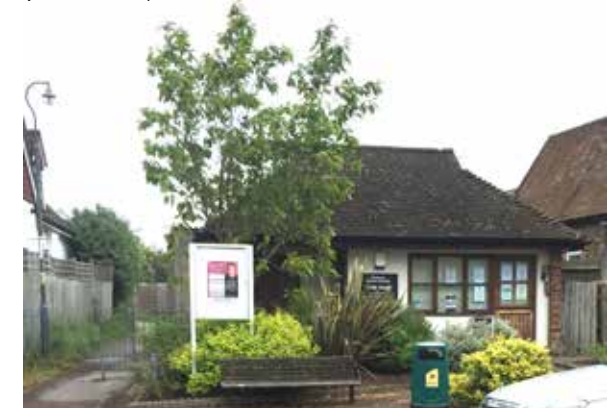
Figure 19: Shenley Parish Council Hub, London Road (24 m 2 gross floor area including accessible public toilet)
