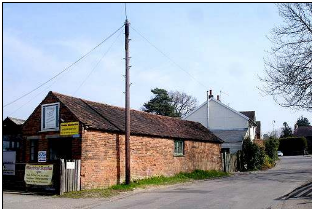
Figure 7. Rectory Lane. Small-scale workshop building retaining link to earlier commercial activity.
