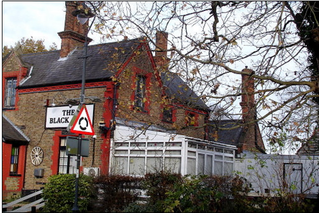
Figure 12. Inappropriate additions to rear of The Black Lion
