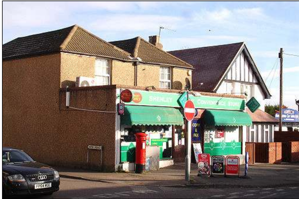
Figure 13. Unattractive shop front
