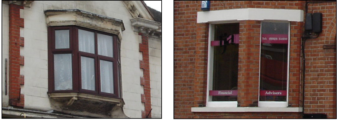
Figure 21. Character Zone 1: loss of traditional architectural features; replaced windows in the High Street
