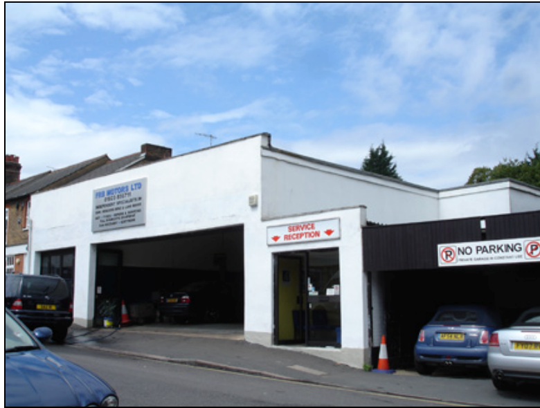
Figure 22. FRB Motors Ltd garage buildings
