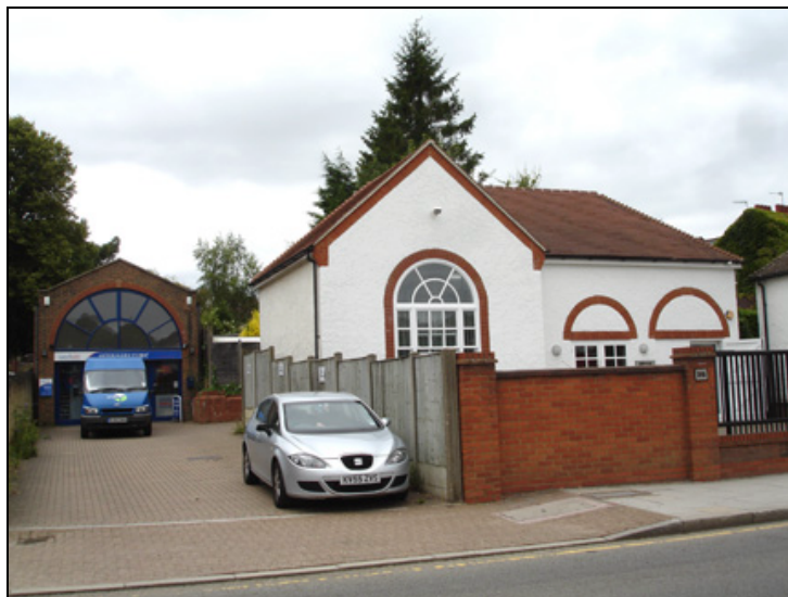
Figure 25. No 34a Watling Street
