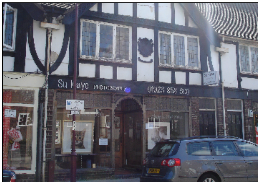
Figure 19. The Oakway – a good example of a little altered carved timber shopfront with appropriately sized fascia sign
