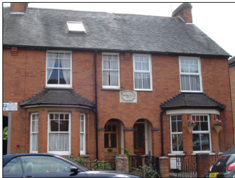
Figure 33. Newland Villas. Original timber sash windows (left) contrasting with uPVC replacement windows in a matching style (right)
