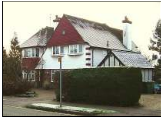
36 Heath Drive; an original 1920s house
