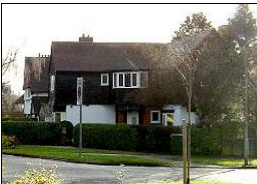
38 Heath Drive, a winged-house type at the island; one of the original 1920s houses
