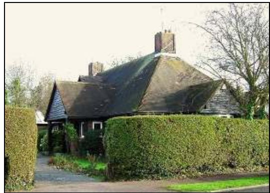
45 Heath Drive; an original 1920s house
