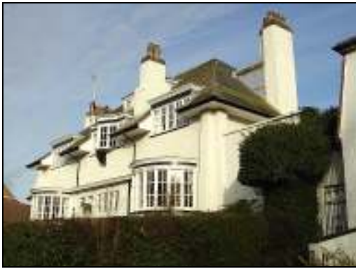
'Seldown' (no. 23) by Sir Banister Fletcher. Listed building. The first house to be erected on the Potters Bar Garden Estate c1903
