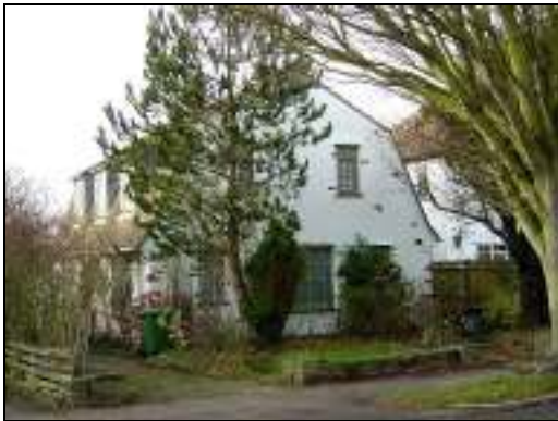
44 Heath Drive; an original 1930s house
