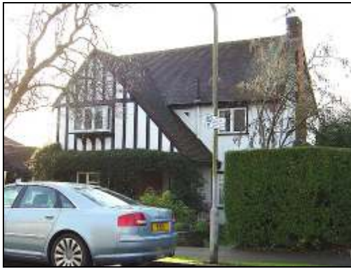
24 Heath Drive; an original 1920s house
