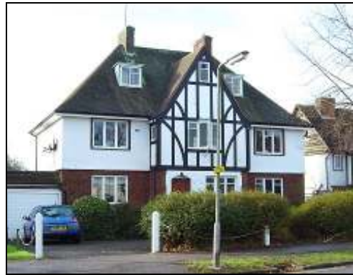
'Homeleigh' (no. 22) originally designed by Sir Banister Fletcher c1909. Demolished by a bomb in 1941 & re-built in the 1950s
