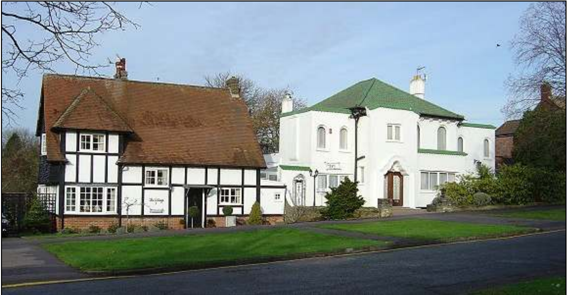
Two of the original houses on Manor Way (west): no. 2 (1920s) and no. 4 (1930s)
