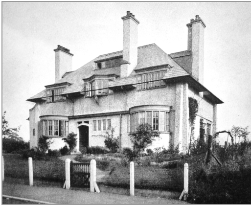
Photograph of Seldown , The Avenue (front)
