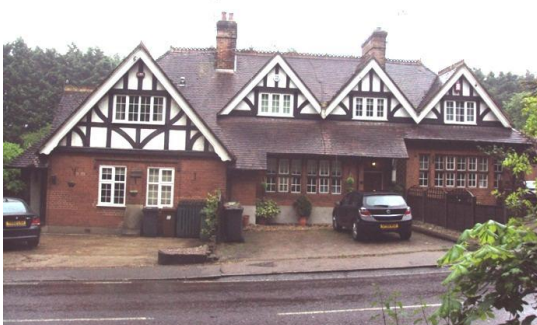
Figure 2: 5-9 Elstree Hill North (Left)
