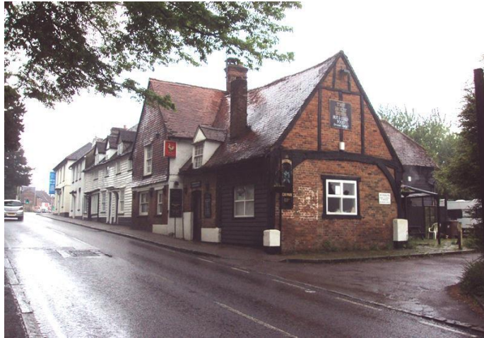
Figure 4: The Holly Bush Inn and cottages, High Street (Above)
