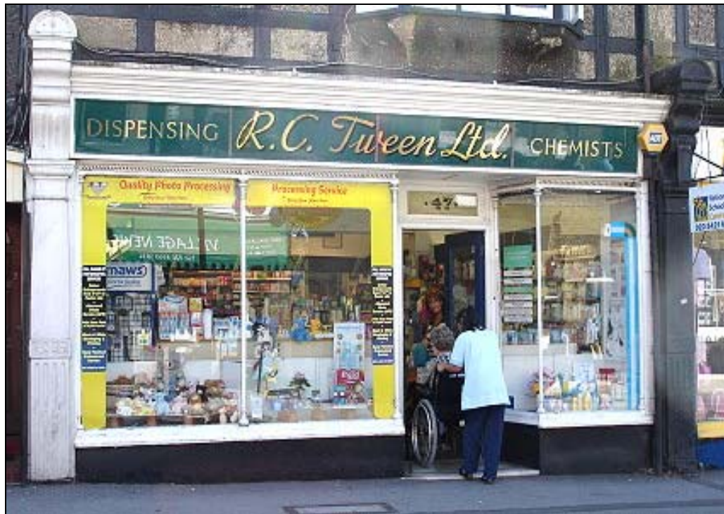
Figure 29. Character Zone 2: a good example of a retained shop front with large display windows, traditional hand painted fascia, pilasters, consoles, stall riser and a recessed doorway with fanlight over (47 High Street)
