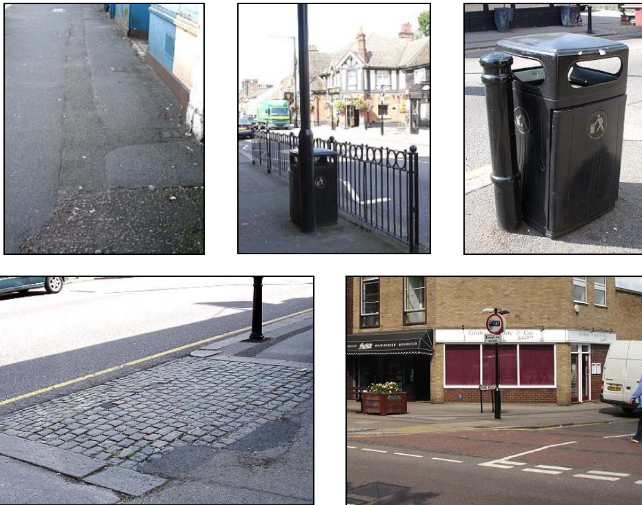
Figure 27. Character Zone 2: negative factors; examples of poor street paving, signage and bins on the High Street
