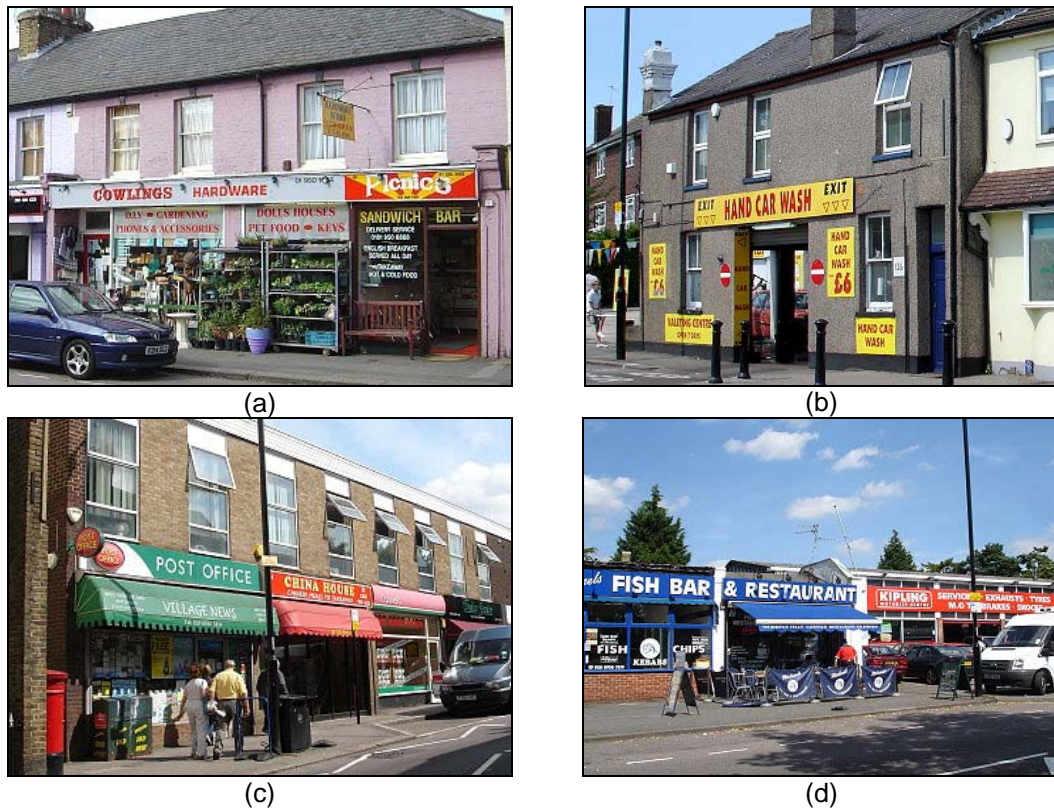
Figure 32. Character Zone 2: negative factors; examples of brightly coloured, multiple and over sized signs and advertisements used along the High Street. Nos. 40 – 42 (a); 134 – 136 (b); 82 – 94 (c); 148 – 152 (d)
