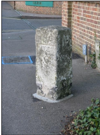
Figure 2 - The Historic Boundary Marker, taken facing north.
