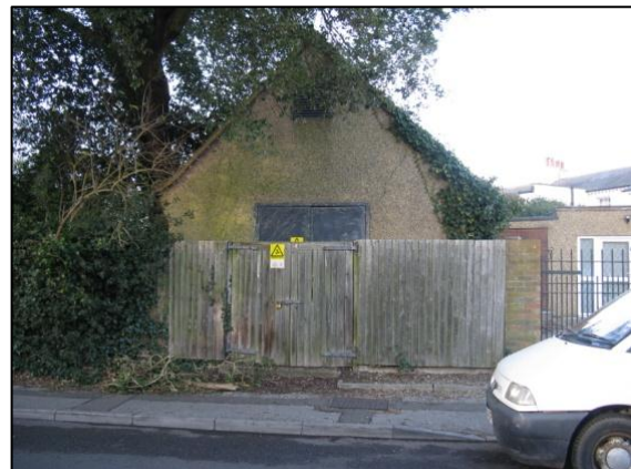
Figure 27 - The electrical substation along Hartsbourne Road.
