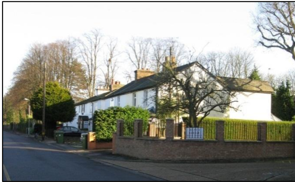
Figure 8 - Nos. 2-16 Windmill Lane
