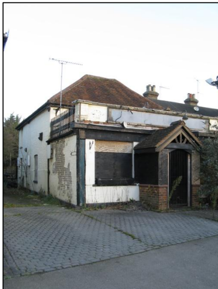
Figure 14 - The Devonshire Arms, now closed and dilapidated.
