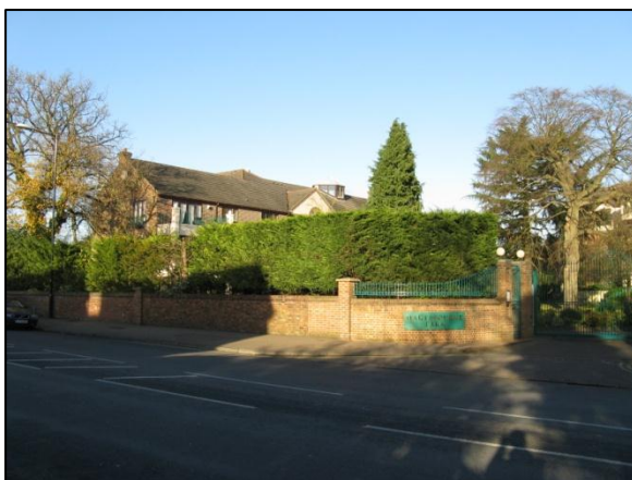
Figure 30 - Hartsbourne Park, looking North East.
