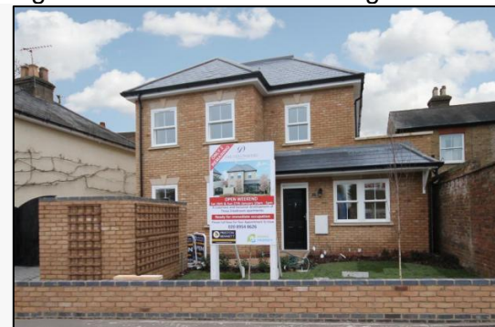
Figure 36 - The new 'Devonshire' development.
