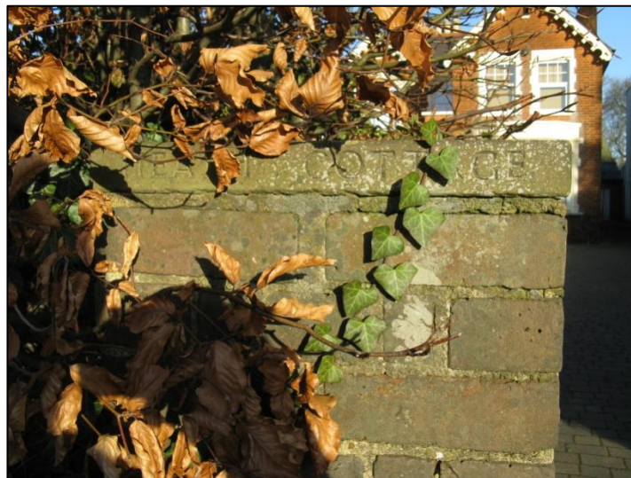
Figure 32 - Capstone of the gatepost at No. 172 High Road.
