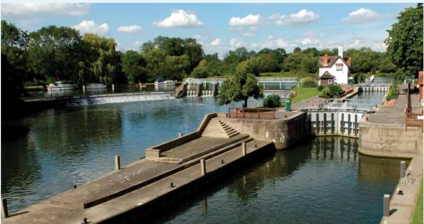
↑ There are 44 lock and weir sites on the River Thames
