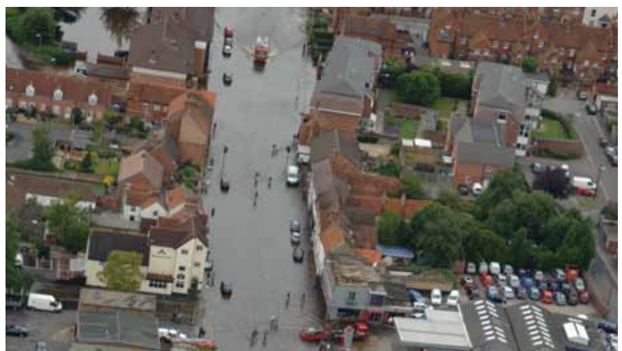
↑ Flooding in Oxford, July 2007.
