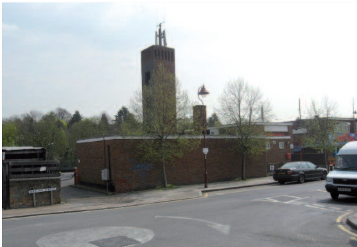
Photograph 2: The former Radlett Fire Station viewed from the west
