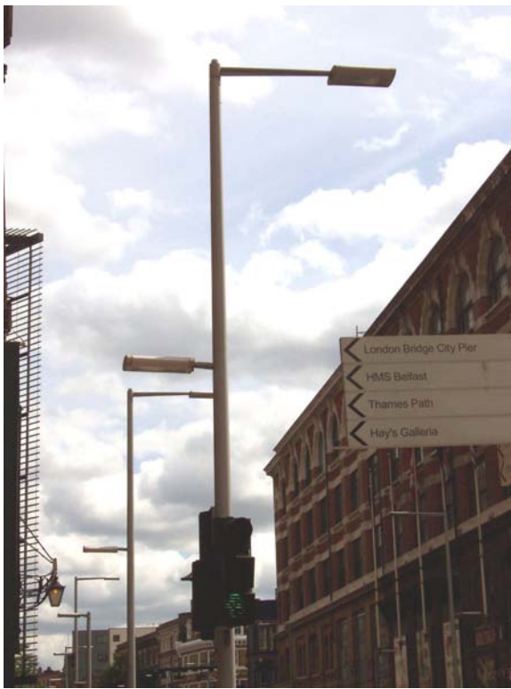
Figure 6.4: Example of combined signal and lamp column
