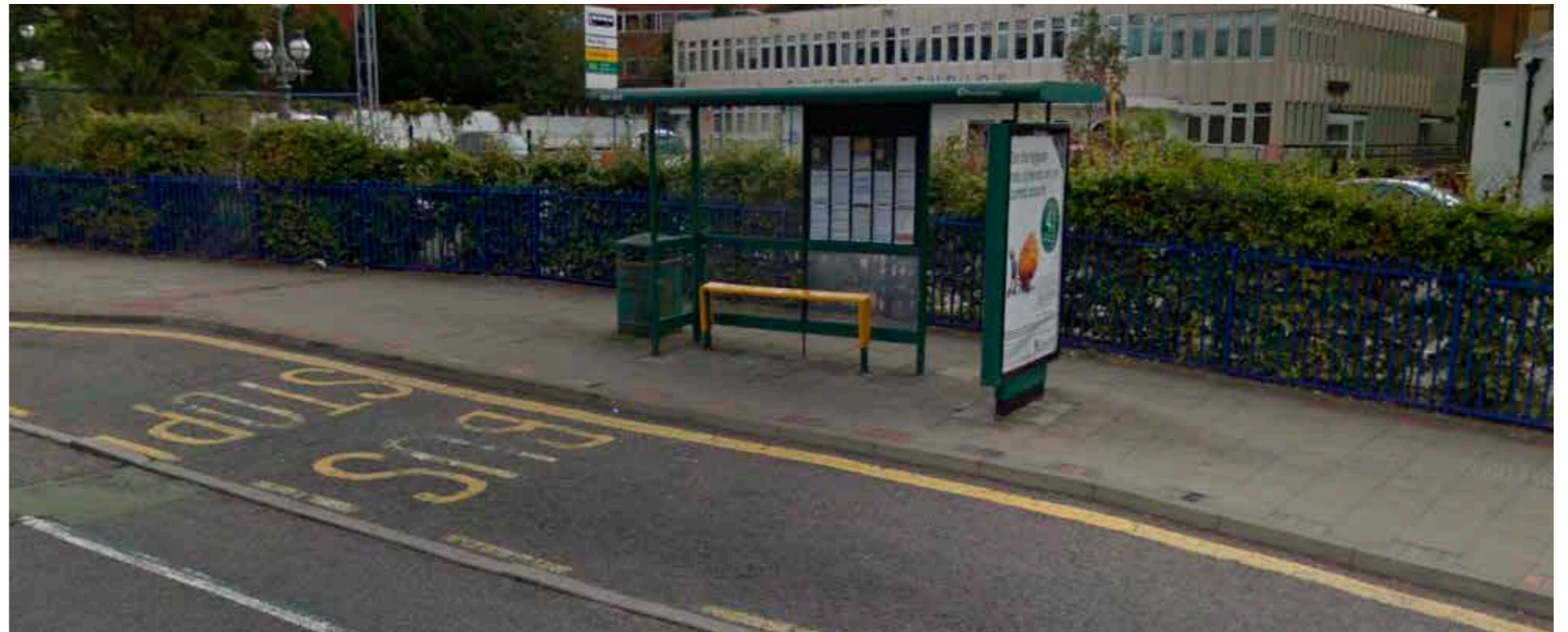
Figure 9 – Non Equality Act compliant bus stop, which also results in delay for buses rejoining traffic.
