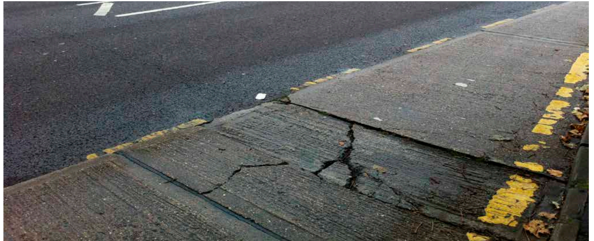
Figure 8 – Existing bus stop on Elstree Way (close to its junction with Studio Way) with poorly maintained concrete surfacing.
