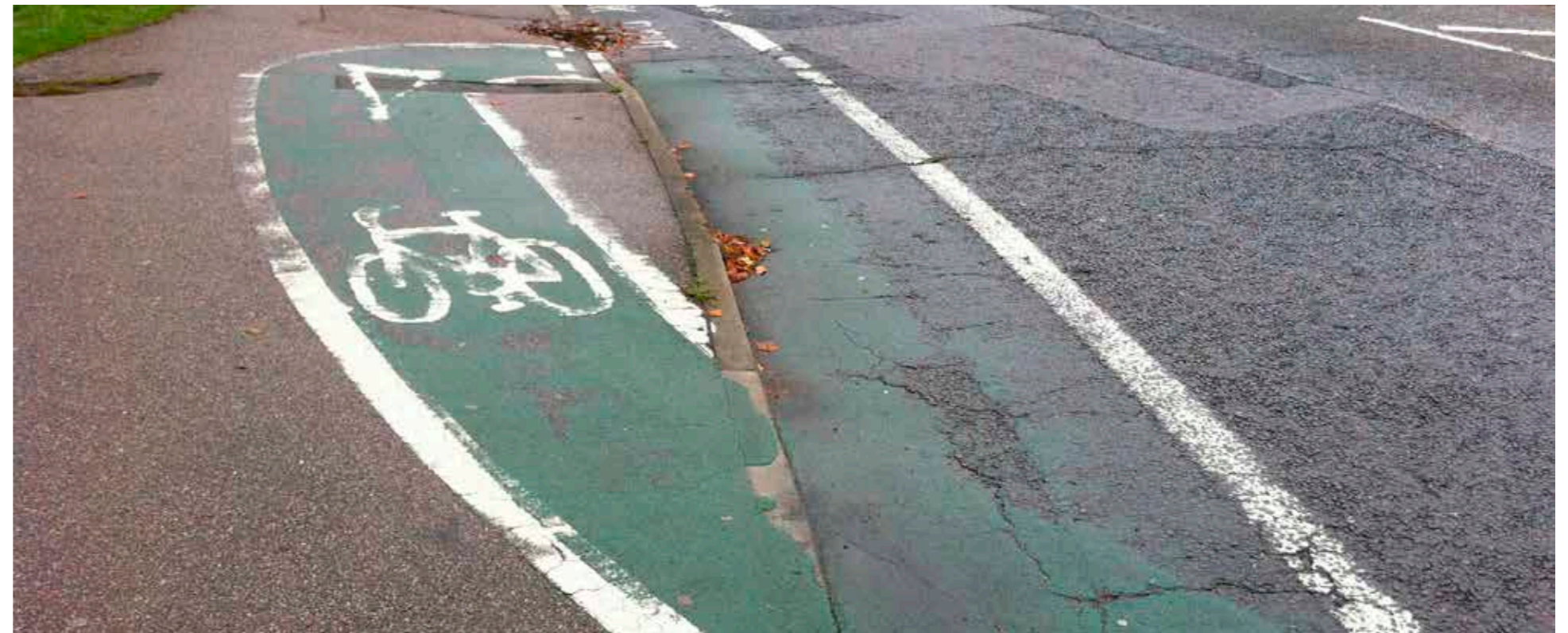
Figure 7 – An example of poor alignment for cycle movements at Elstree Way/ Shenley Road roundabout.
