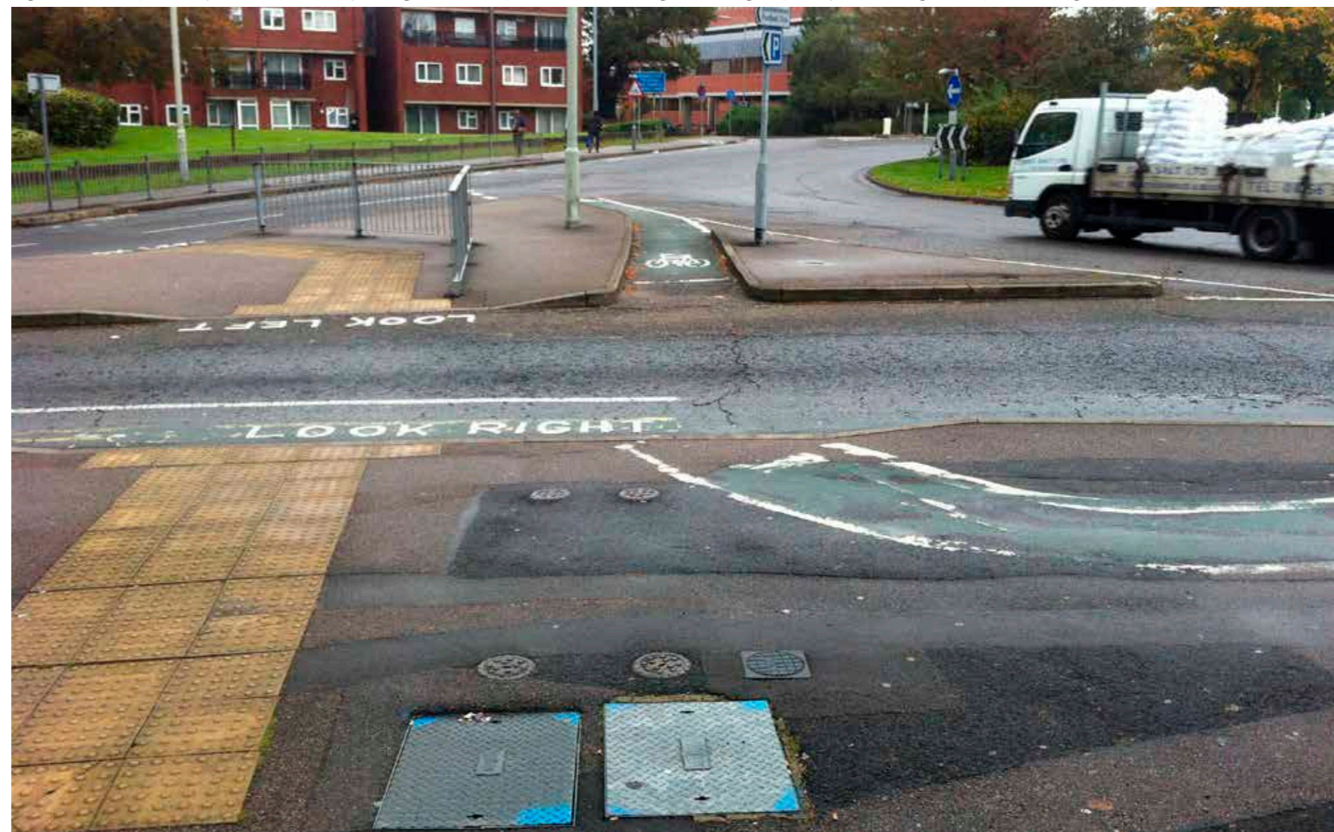
Figure 3 – Poor cycle and pedestrian facility, poor sight lines for cyclists when entering the carriageway and poor existing footway and carriageway surface.
