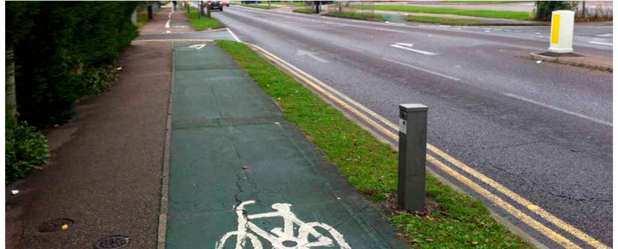
Figure 6 – Uneven surface with lack of coloured in-fill on existing cycle tracks.
