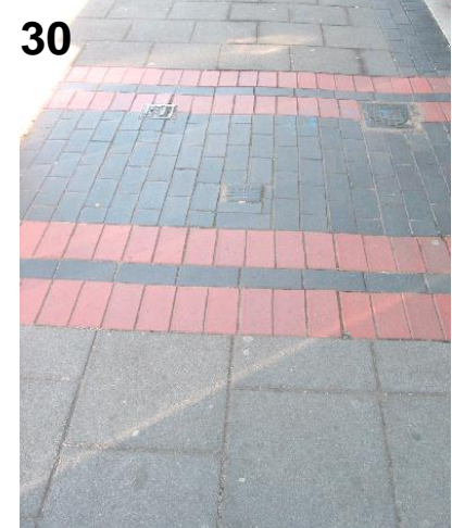
30. The paving stones in the foreground are not in line, where the slabs have been laid vertically rather than horizontally as at the top of the picture (Borehamwood).
