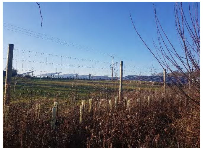
54B/a: Potters Bar Fringe showing solar panels adjacent to railway line
