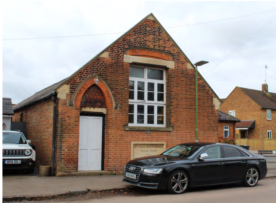
Figure 35 South Mimms Village Hall (Parish Rooms)
