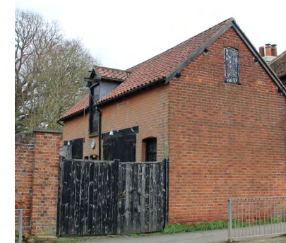
Figure 26 Former Vicarage stable and cartshed
