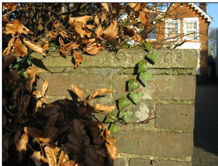
Figure 32 - Capstone of the gatepost at No. 172 High Road.
