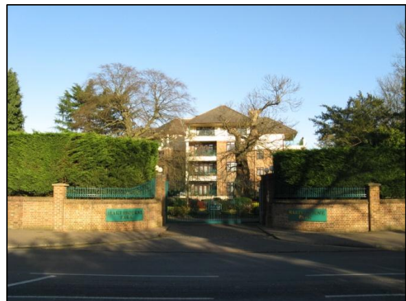
Figure 31 - The main entrance of Hartsbourne Park
