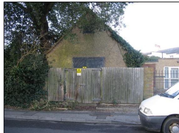
Figure 27 - The electrical substation along Hartsbourne Road.
