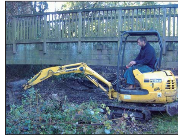
Excavating the moat
