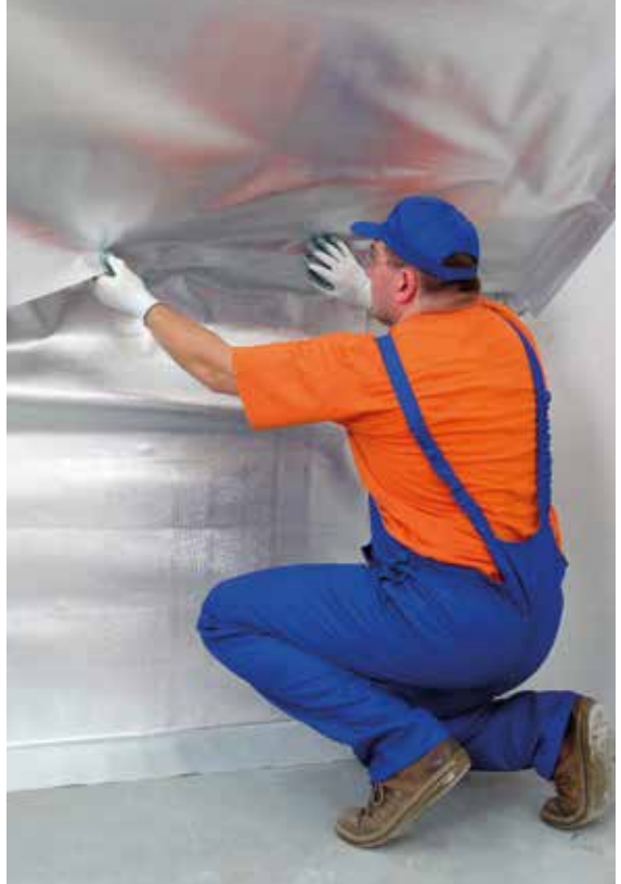
Fitting vapour insulation foil under thermally insulated attic surface
