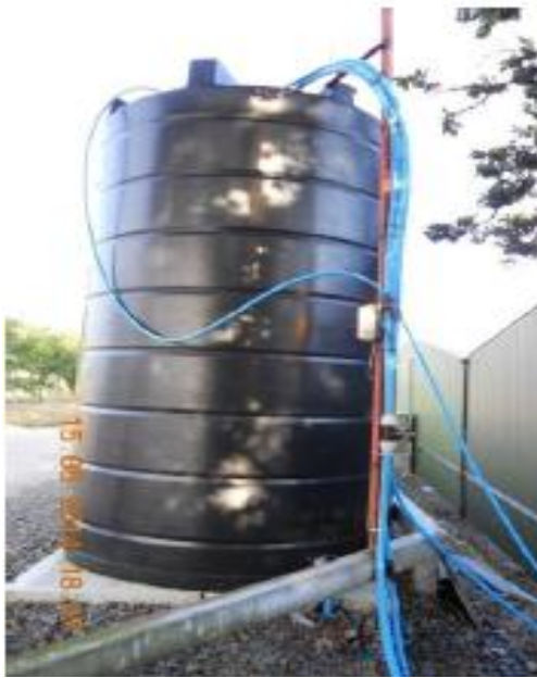
Figure 21: Tanks in which mains water and borehole water were blended and stored
