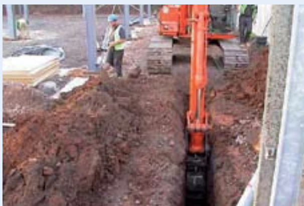
Stage 1: Excavate a trench, making sure that all the knotweed is contained.
